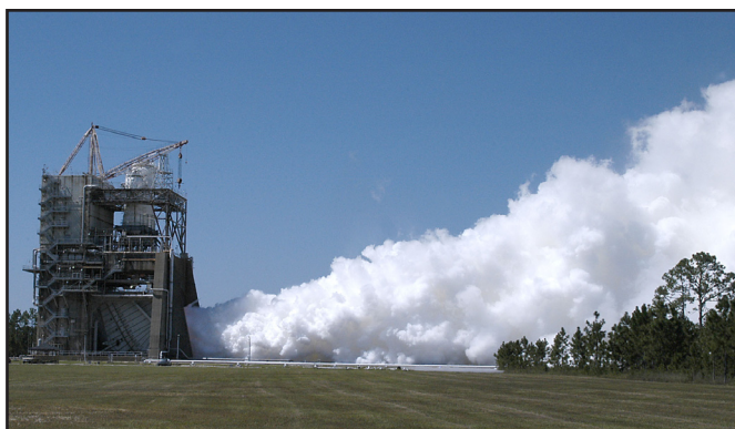
SSC's A-1 Test Stand, site of the first space shuttle main engine test in 1975, conducted its final space shuttle main engine test in 2006. A-1 then began a new chapter in its legacy: conversion to testing J-2X engines, which will power the upper stage of NASA's new crew launch vehicle, the Ares I.
